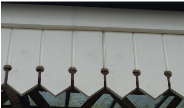
After Replacement - POLYboard Dagger Boards
