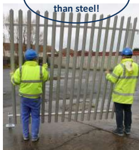
Fitting the panel
